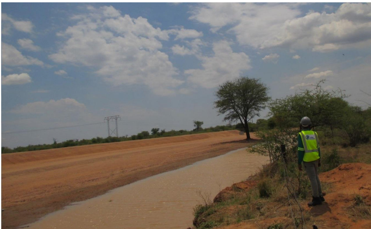
Figure 13: Unlined clean water diversion channel at Medupi
