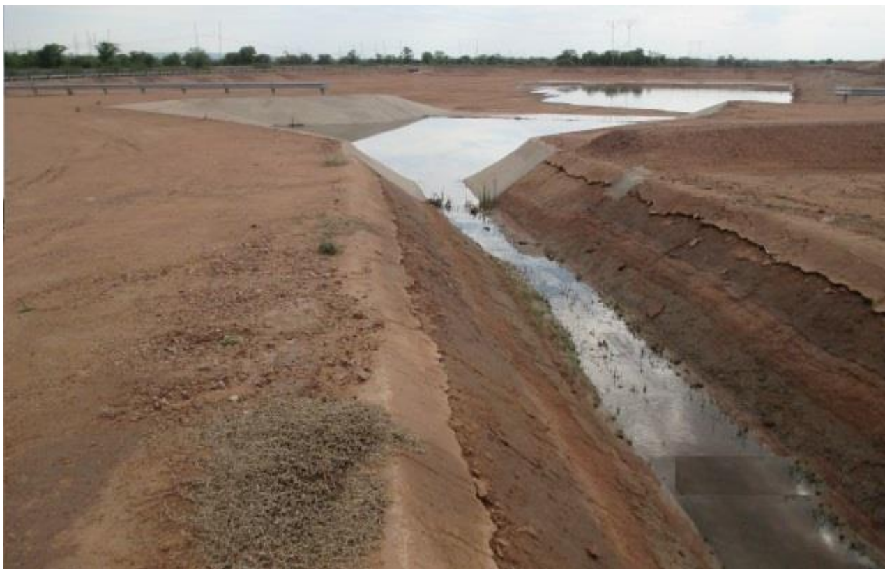
Figure 12: Concrete-lined dirty water containment channel draining into PCD at Medupi
